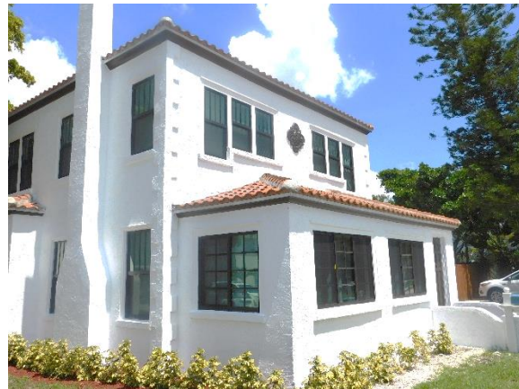
Example: 331 South Federal Highway After: Aluminum Single-Hung and Horizontal Rollers Replacement Windows
