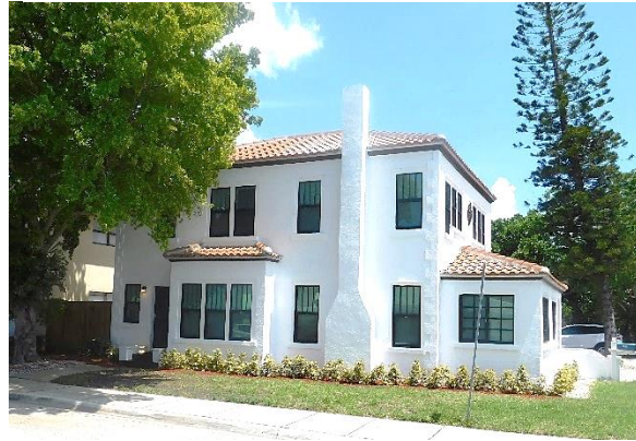
Example: 331 South Federal Highway Aluminum Single-Hung and Horizontal Rollers Replacement Windows (Administrative Approval)
