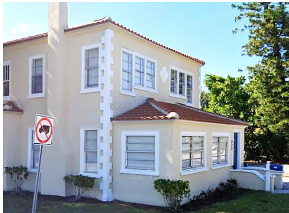
Example: 331 South Federal Highway Before: Mixture of original wood double-hung windows and replacement awning windows
